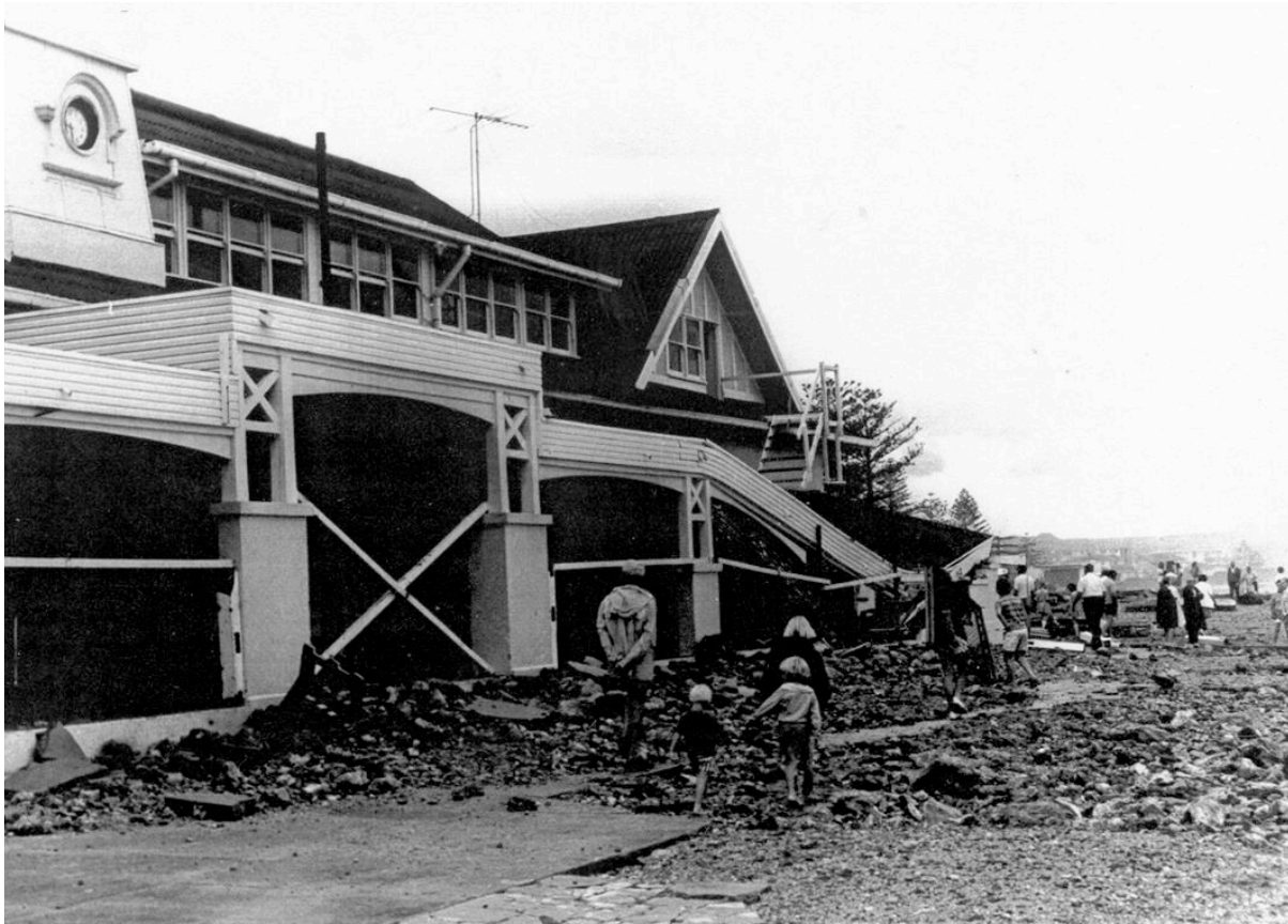
Figure 4 Wave and storm surge damage caused by Pam at Kirra.
