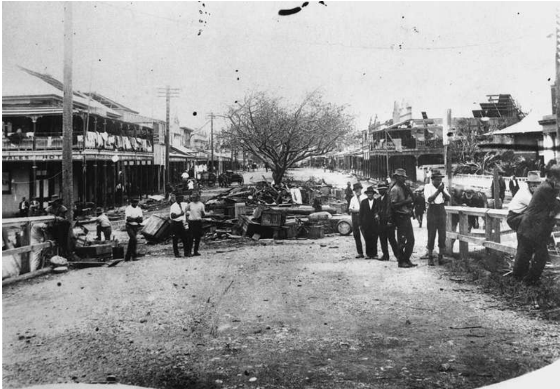
Looking south down Sydney Street after a cyclone in Mackay in 1918. Many unroofed buildings and debris are visible in the street with trees having been stripped of their leaves. Clothing is hanging over the verandah railings to dry.
