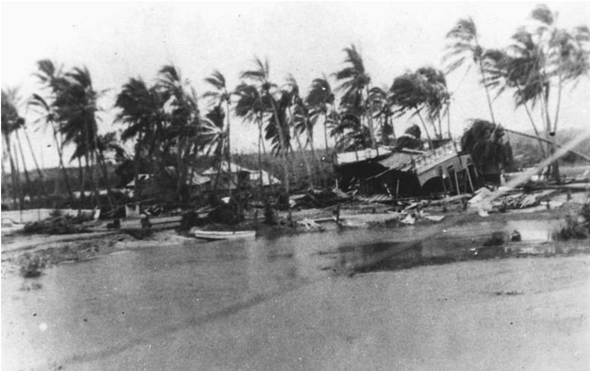
Cyclone damage at the Pioneer River, Mackay, 1918 contributed by QldPics taken in 1918
